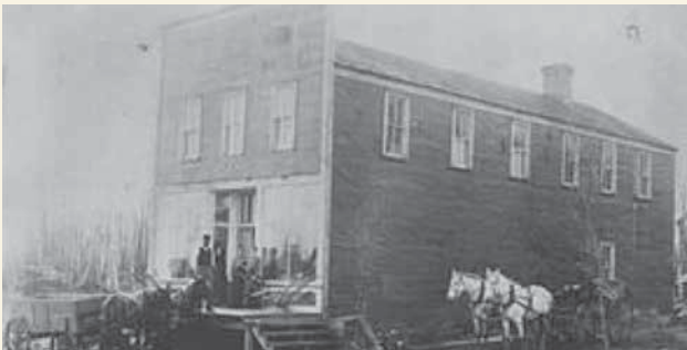
E.W. Leeper Store northeast of Erhard
