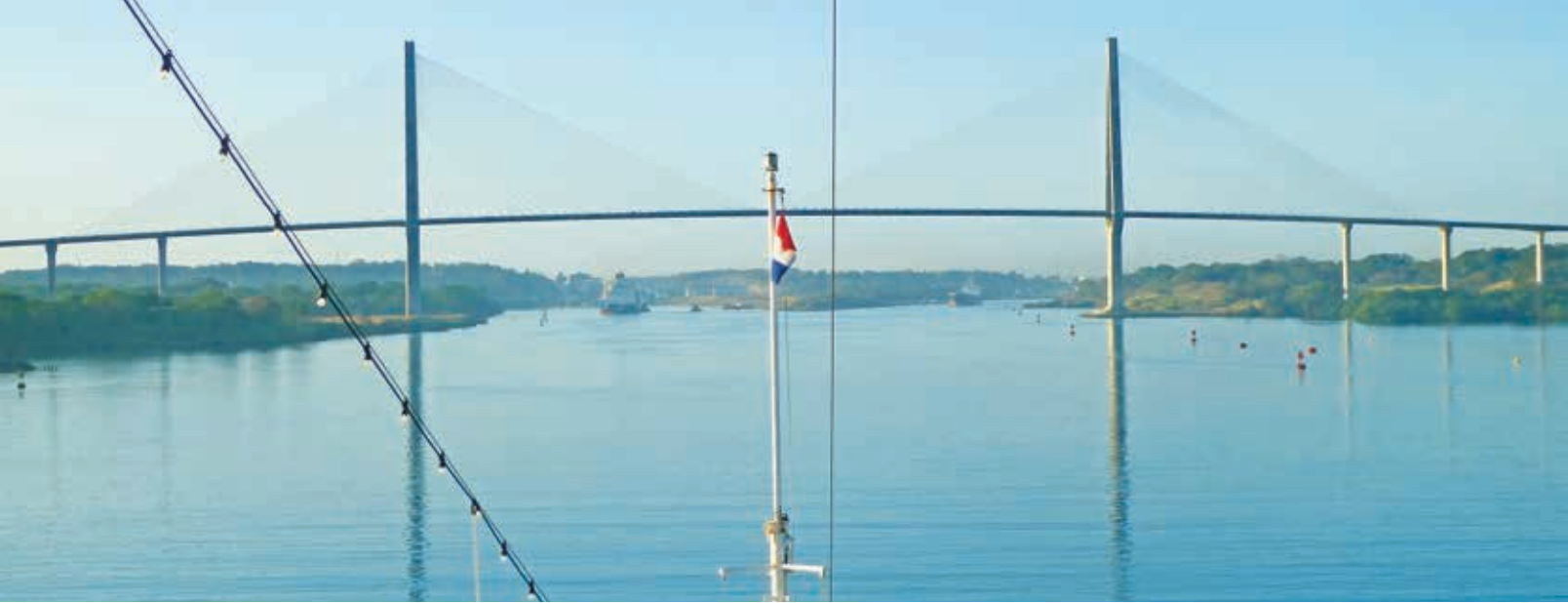
Atlantic Bridge at Panama Canal, Colon, Panama
